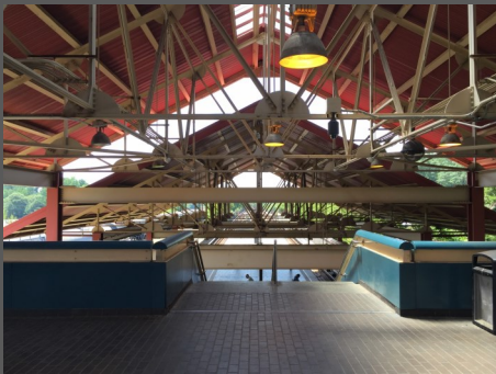
Inside the station
